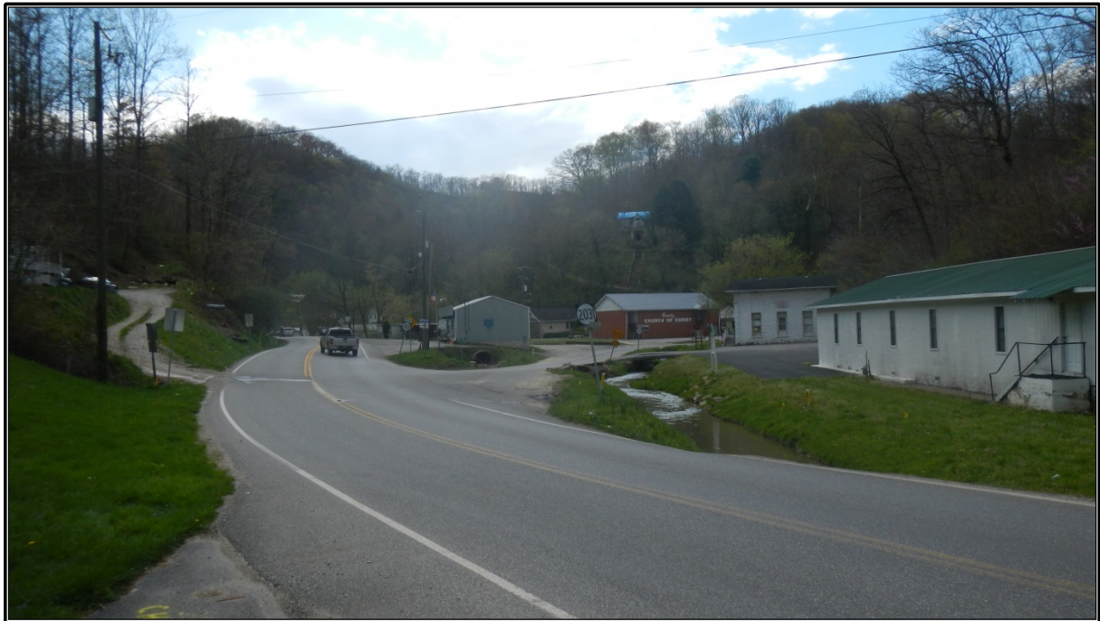
Figure 4. General overview showing manicured lawns in and around the junction, facing west.
